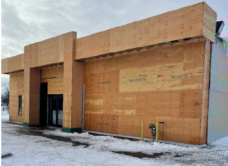
Photograph 5 - Front of commercial business adjacent south of the Site (formerly Kilby's Auto, now TruckTown) at 5831 Perth Street.
