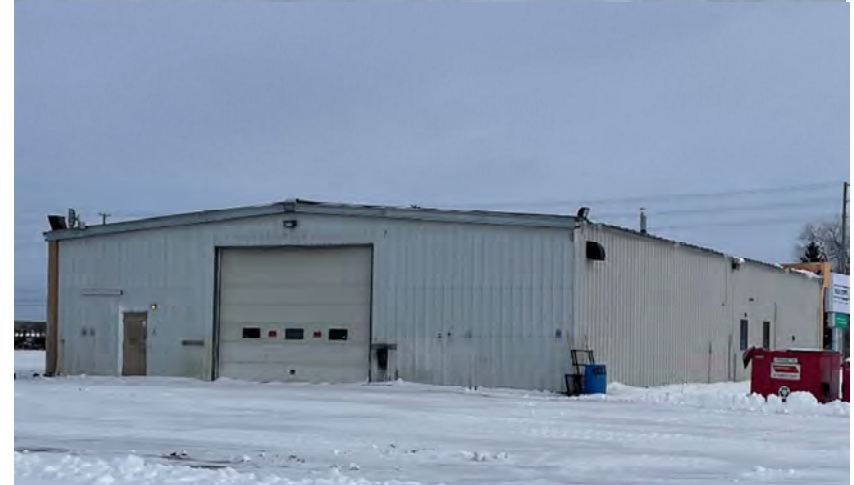
Photograph 6 – Vacant parking lot and rear of building at 5831 Perth Street.
