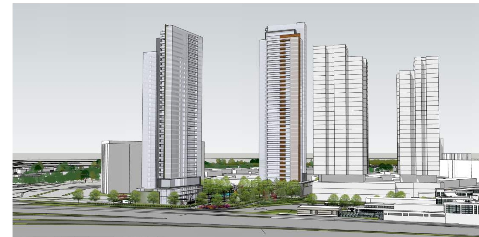
2. View from SE / Highway 417 Westbound
