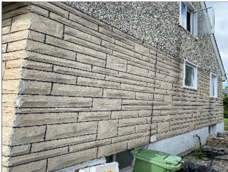
Photo 6 – Site Building C (northeast elevation).
