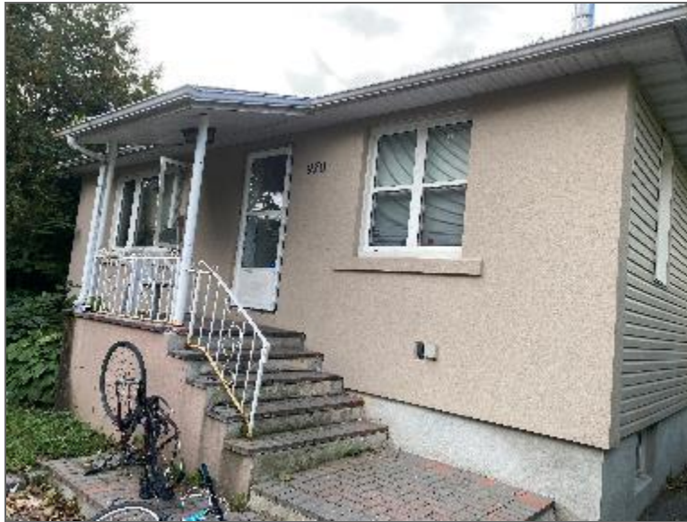
Photo 1 – Site Building A (northeast elevation).
