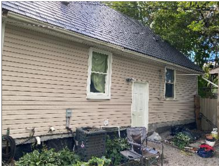
Photo 8 – Site Building D (northeast elevation).
