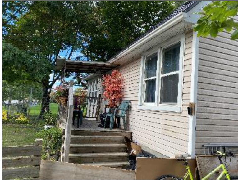
Photo 7 – Site Building D (southeast elevation).
