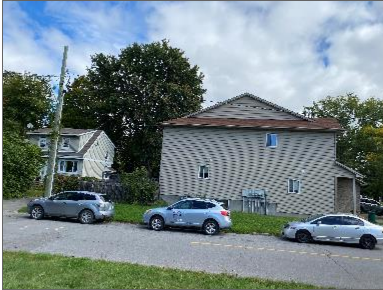
Photo 11 – Properties located northeast of the Phase One Property.
