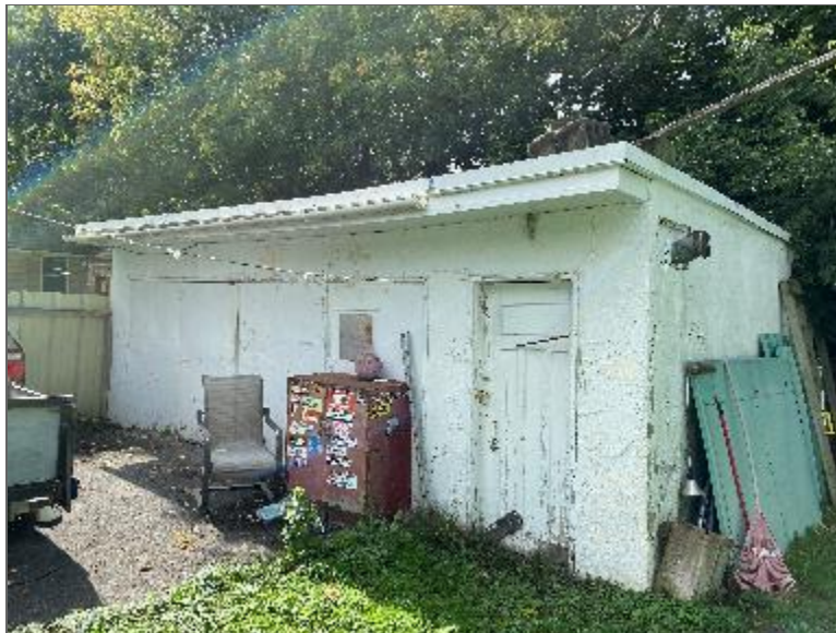
Photo 4 – Storage shed located southwest of Site Building B.
