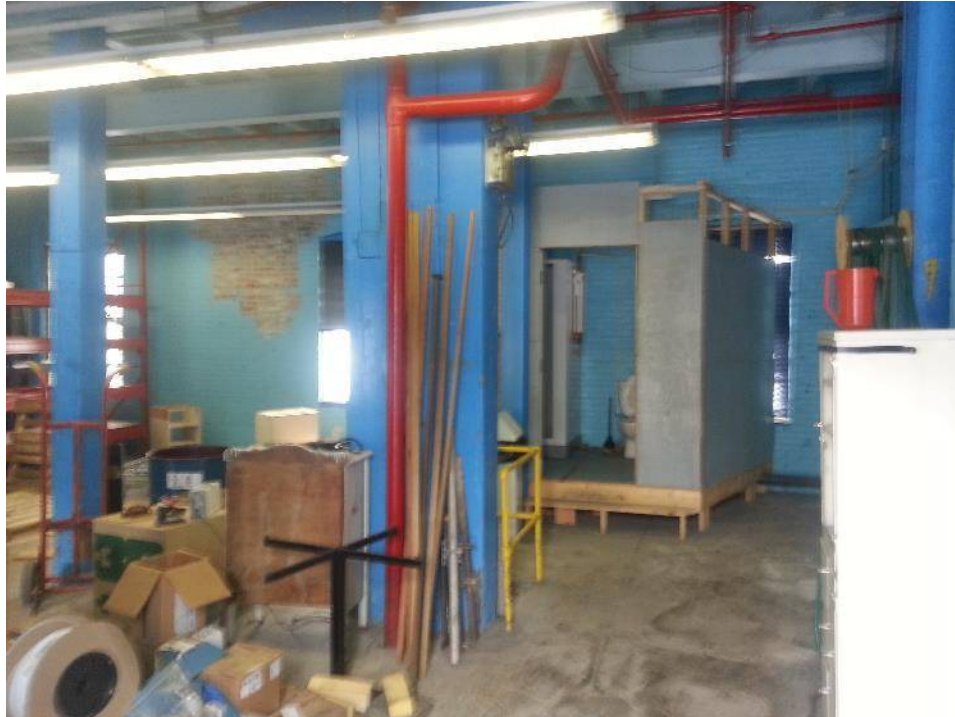
Photograph 5: View of interior of Building 542, facing south (April 7, 2014)
