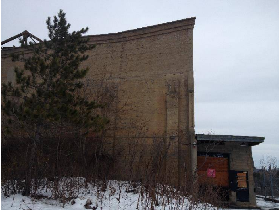
Photograph 3: View of west side of Buildings 534 and 534a, facing east (April 7, 2014)
