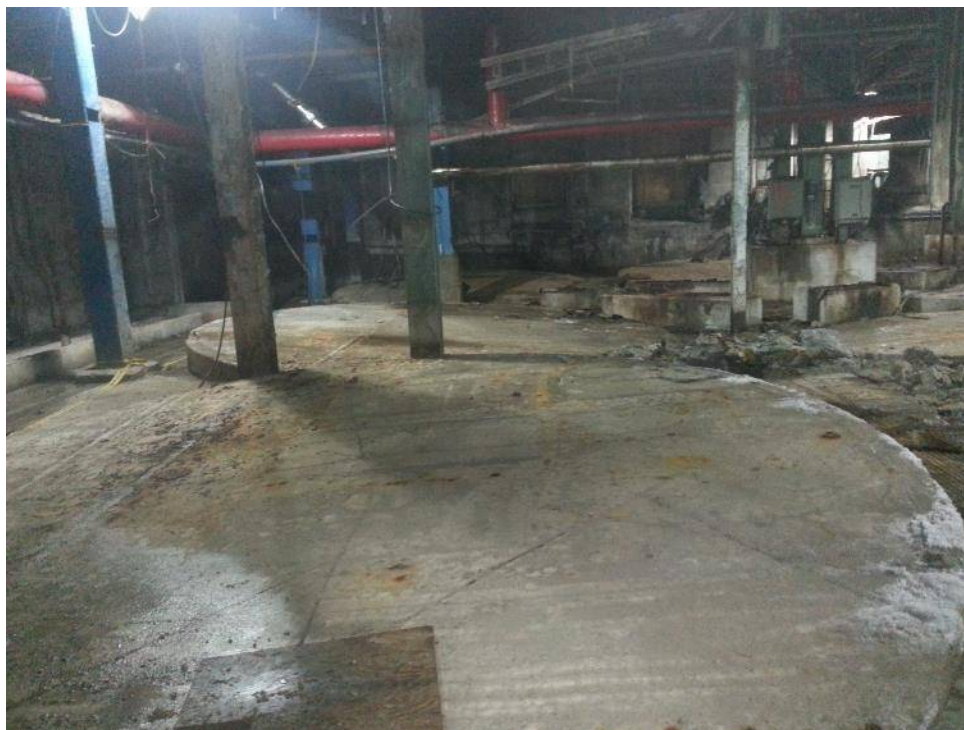
Photograph 10: View of interior of Building 530, facing south (April 7, 2014)
