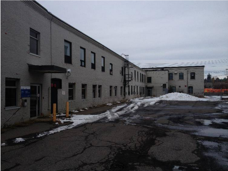
Photograph 2: View of south side of Building 541 and west side of Building 540, facing east (April 7, 2014)
