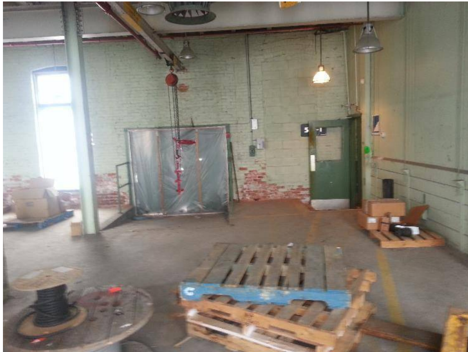
Photograph 6: View of interior of Building 543, facing south (April 7, 2014)
