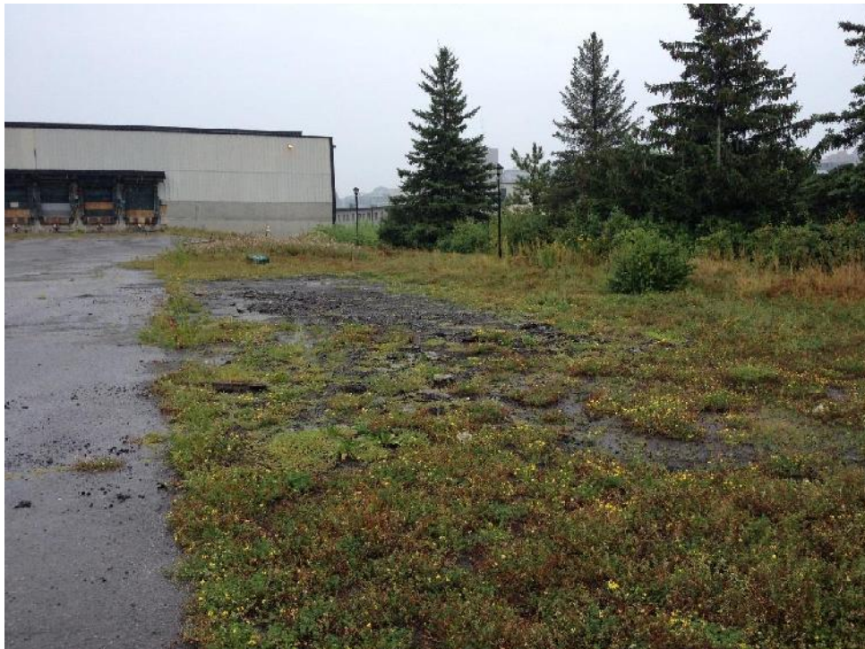
Photograph 14: Ground covered by granular fill material west of Building # 504. Sparse vegetation is visible. Photo taken facing east (August 12, 2014).
