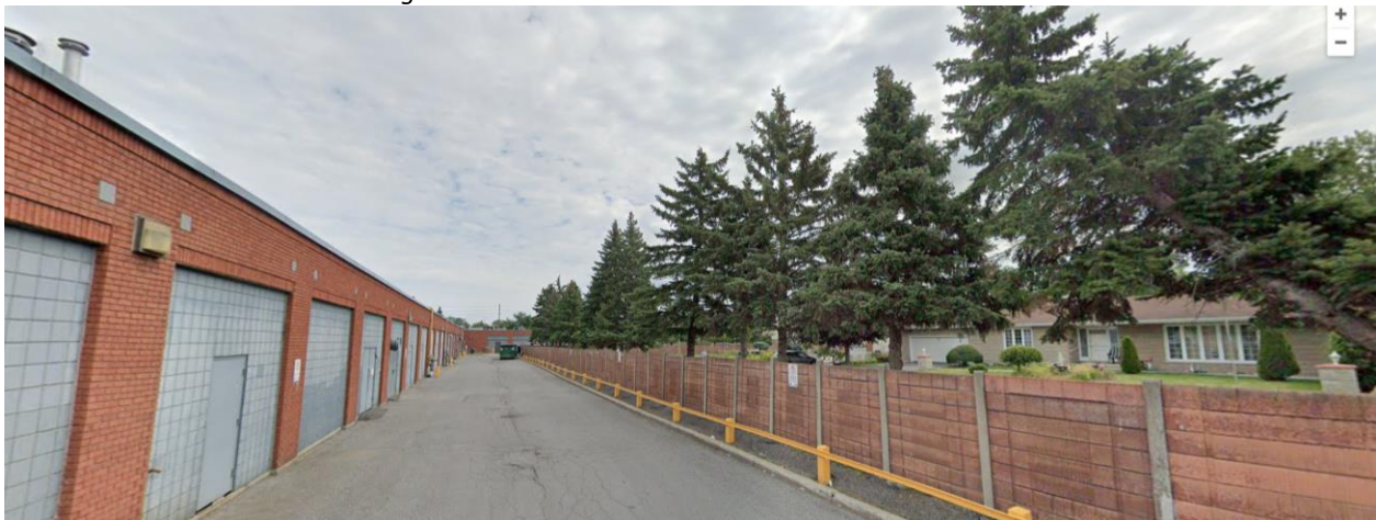
Figure 6: View along the service lane at the rear of the property residential homes along Sunnycrest Drive are separated by a board fence. Source: Google Earth
