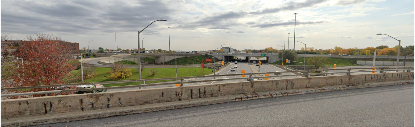
Figure 9: View Looking South from Labelle Street Overpass
