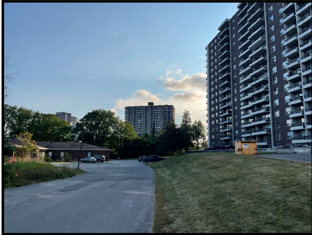
Figure 1: Overview of entrance road and artificial slope up to adjacent property (MH1043-D01).
