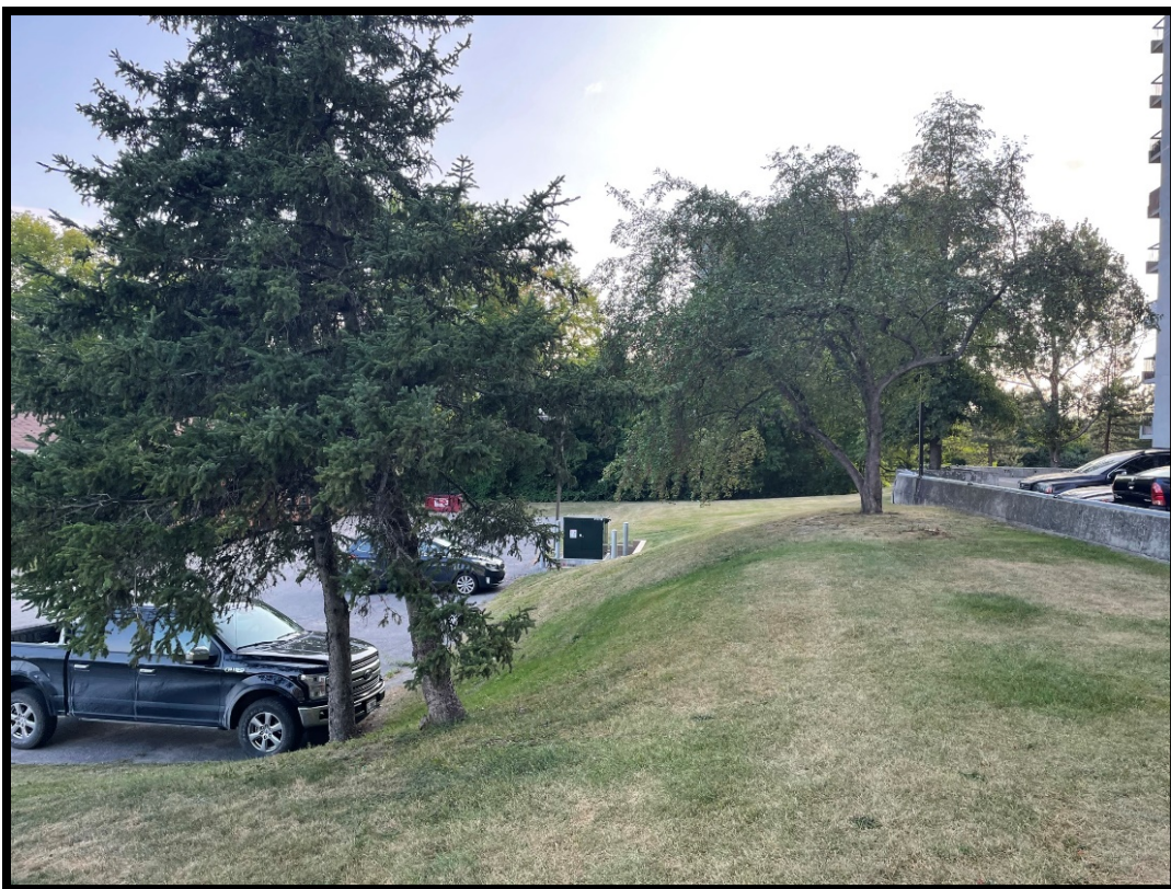
Figure 6: Artificial sloped area and retaining fall south of long-term care facility parking lot with infrastructure (MH1043-D05).
