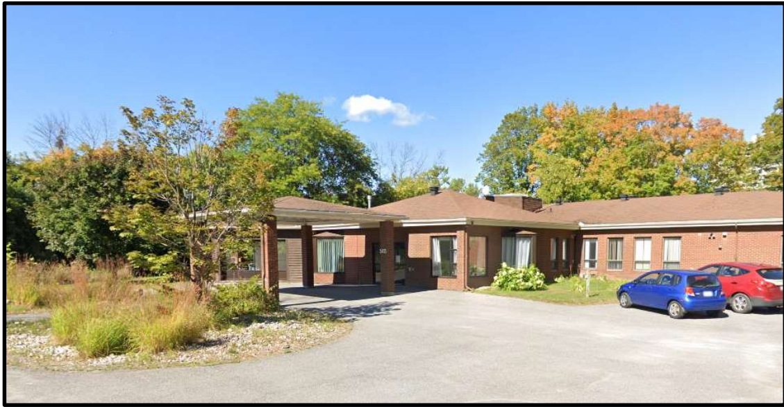
Photograph 1: View of long-term care home looking northeast.
