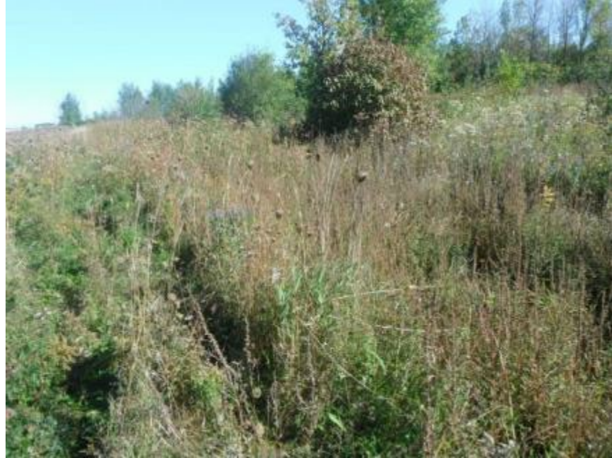
Photo 12: Drain 10 (Station 12) looking upstream from the downstream end (September 17, 2013)
