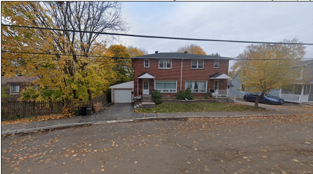
Figure 4. Land uses south of Subject Property
