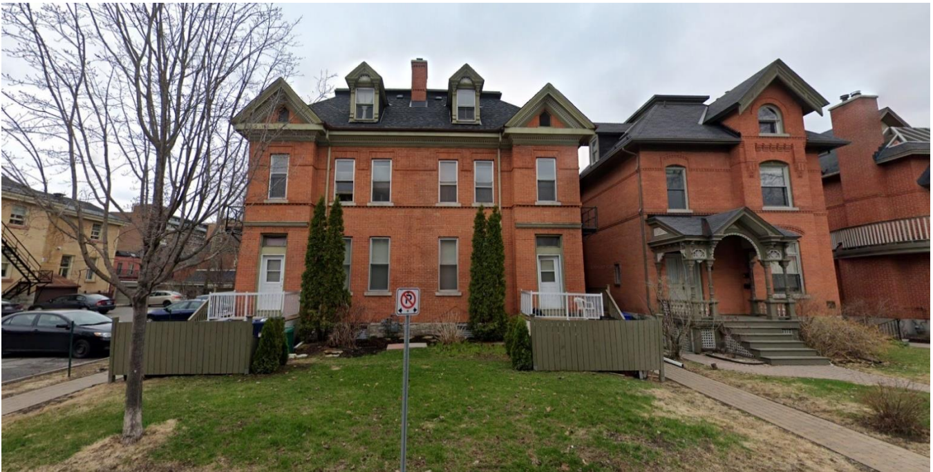
Figure 1: Subject Property frontage on Russell Avenue.
