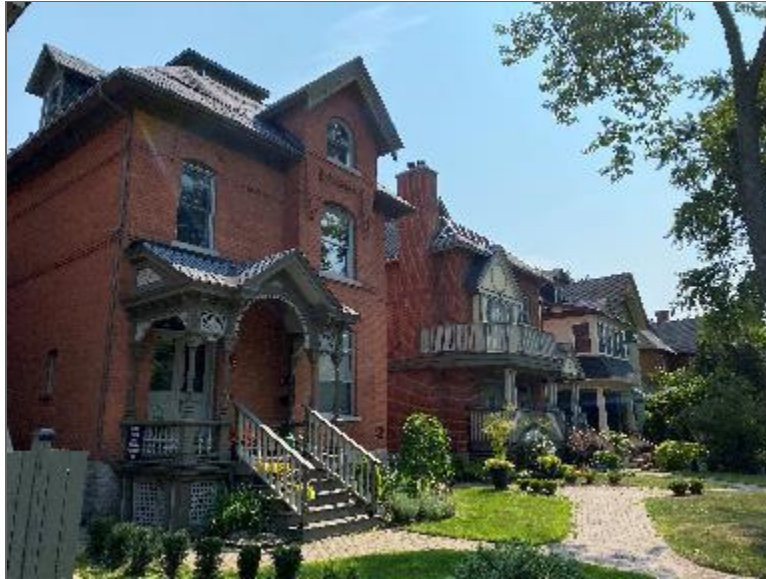
Photo 5 – Properties located southeast of the Phase One Property.
