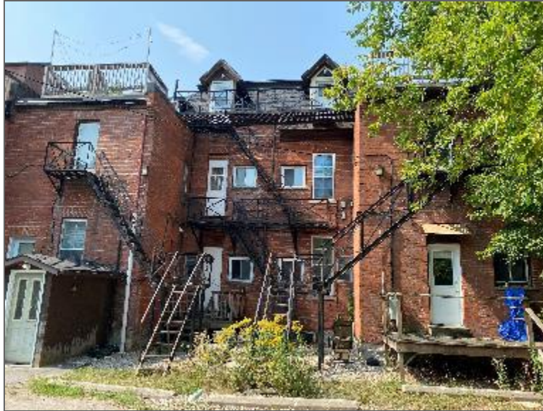
Photo 1 – Site Building (northeast elevation).
