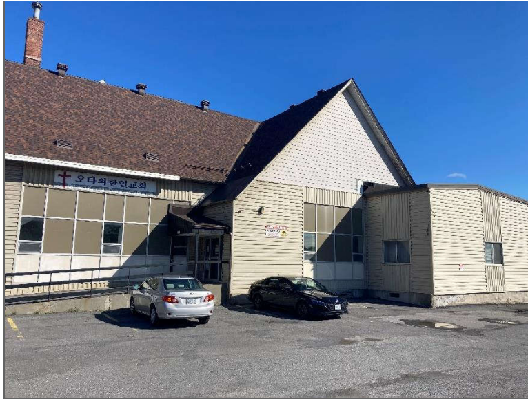
Photo 3 – Site Building (south elevation).
