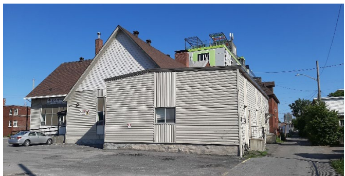
Figure 2: The rear (southern) portion of the church is proposed to be demolished
