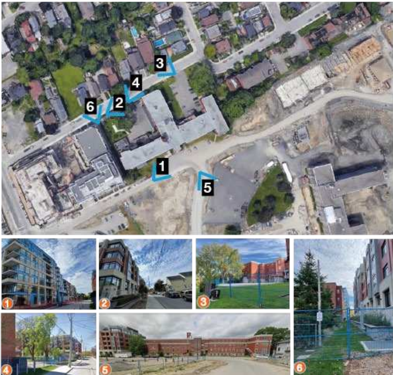
Figure 2. Images of the subject property and surrounding area
