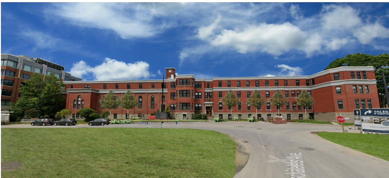
Figure 16. View from des Oblats Avenue
