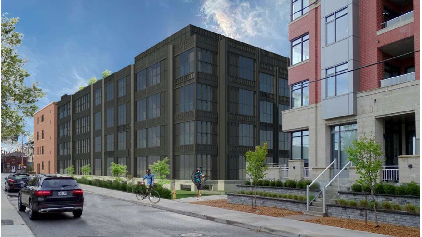
Figure 14. View along Springhurst Avenue from the northwest
