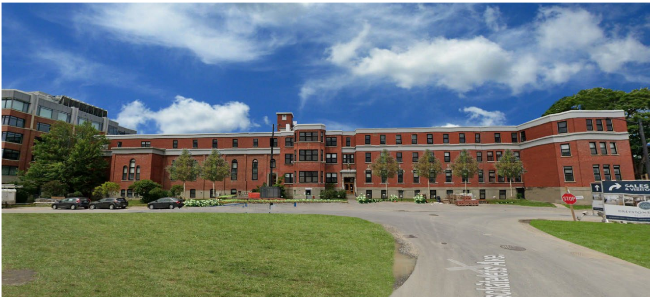
Figure 16. View from des Oblats Avenue
