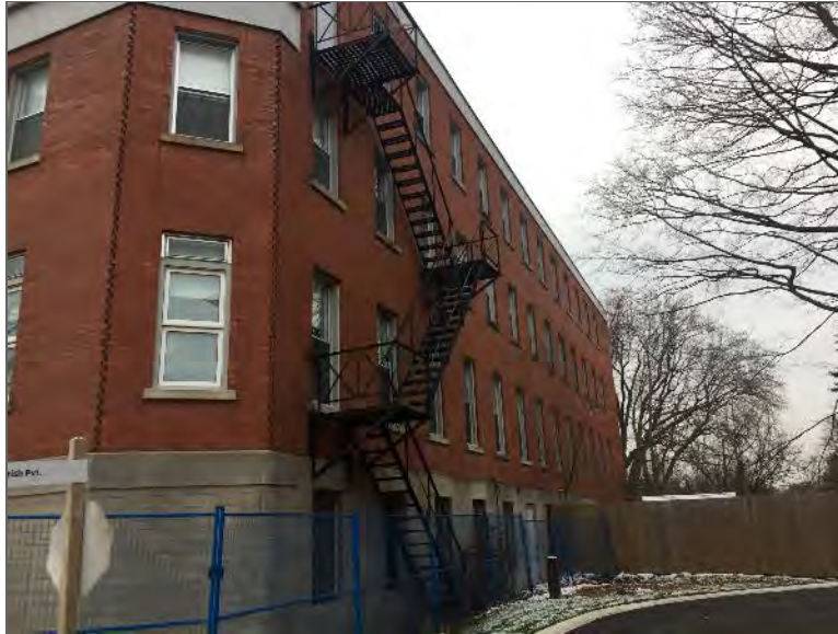
Photo 3 – Site Building (east elevation).
