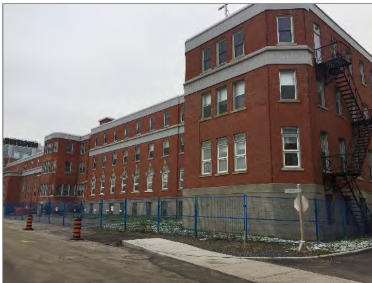
Photo 2 – Site Building (south elevation).
