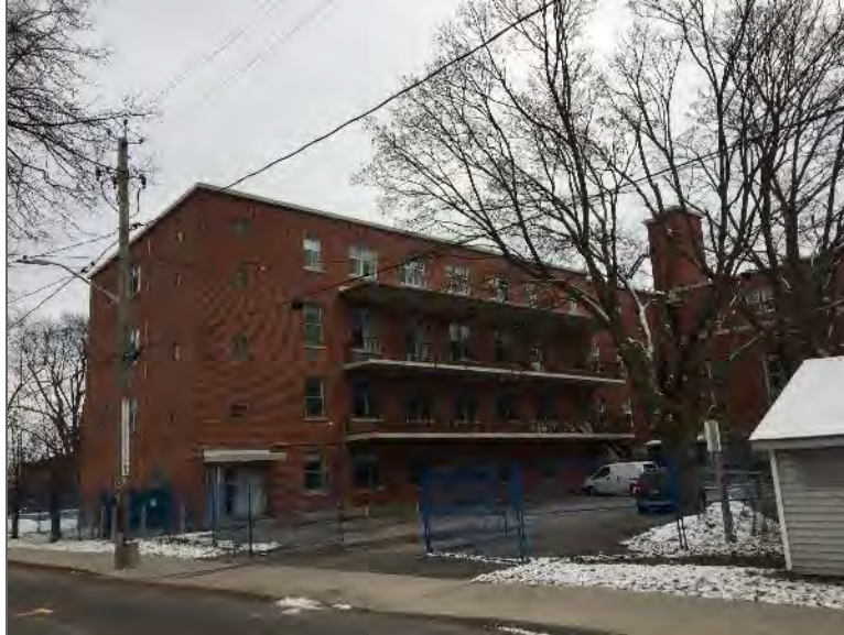
Photo 1 – Site Building (north elevation).
