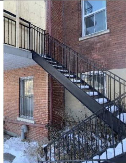
Figure 9: Staircase / Fire Exit from exterior balconies
