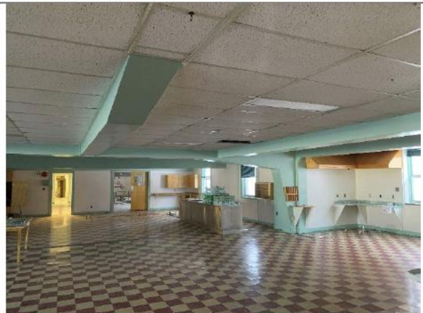
Figure 42: Previous kitchen / dining hall
