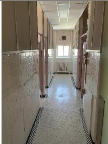
Figure 35: Bathroom Hallway – Women's
