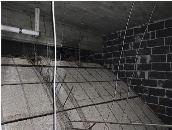
Figure 41: Ceiling cavity. Arch over chancel
