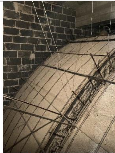
Figure 40: Ceiling cavity. Arch over chancel
