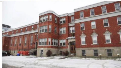
Figure 2: View of main entrance
