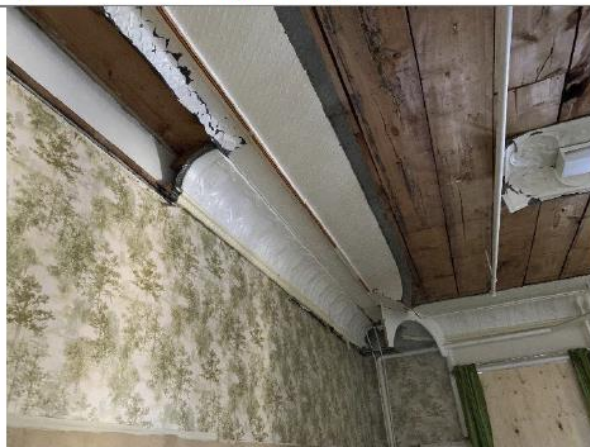
Figure 24: Stripped ceiling finishes
