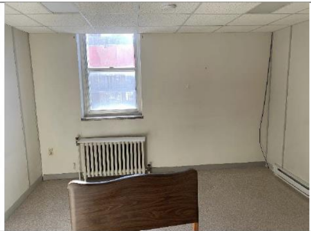
Figure 44: Empty office with sash window
