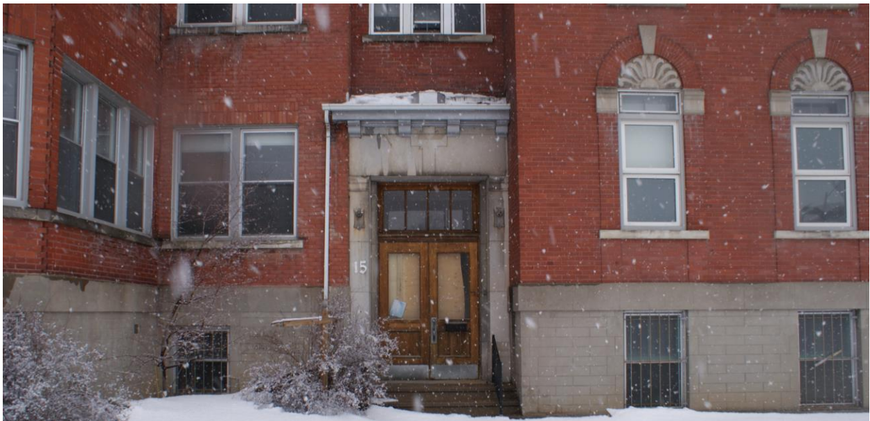
Figure 6: View of the east entrance on the south façade and decorative masonry window detailing on the 1940 addition. The exterior wall of the 1914 structure is to the left of the entrance. The entrance is being retained as part of the rehabilitation with modifications to meet accessibility requirements. Source: Commonwealth
