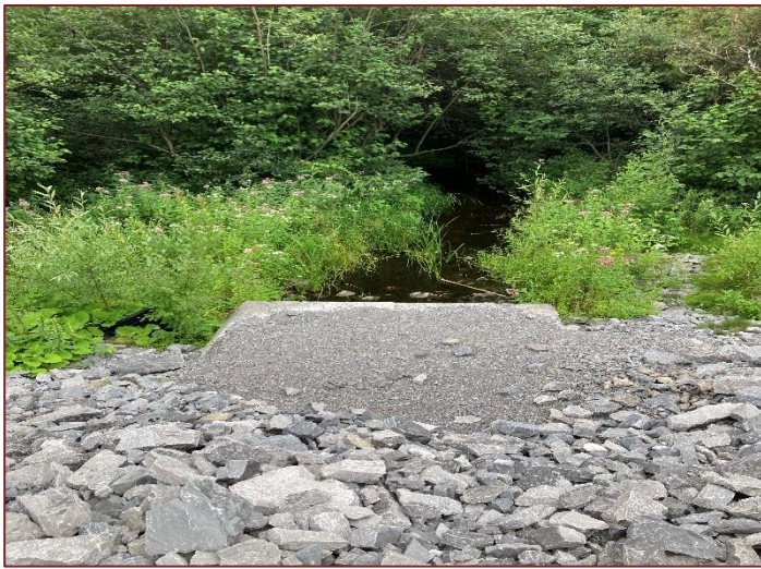
Photograph 5: Unnamed creek flowing through a culvert directly west of the Site under Albert Boyd Road.
