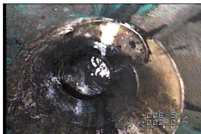
Figure#5: A view to the 75mm 1 o'clock connection to the washroom toilet line at 2.0 meters from the top STACKCO
