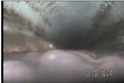
Figure#15: Abandoned due to debris under the murky water and debris sediment at 21.2 meters from the stack
