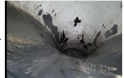
Figure#8: A view to the line deviation downwards at 11.8 meters from the top of MHSA1.
