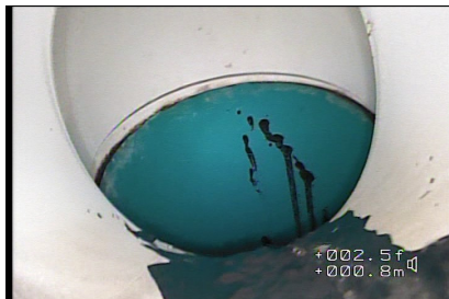
Figure#5: A view to the 75mm 1 o'clock connection to the washroom toilet line at 2.0 meters from the top STACKCO
