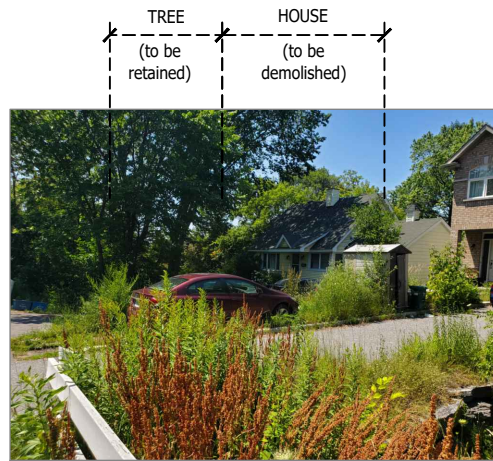
view looking west at property
