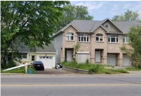
Figure 2-4 Townhouse dwellings east of the site
