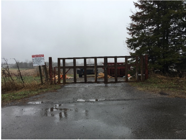
Photo 1: Site access road, located off Old Prescott Road
