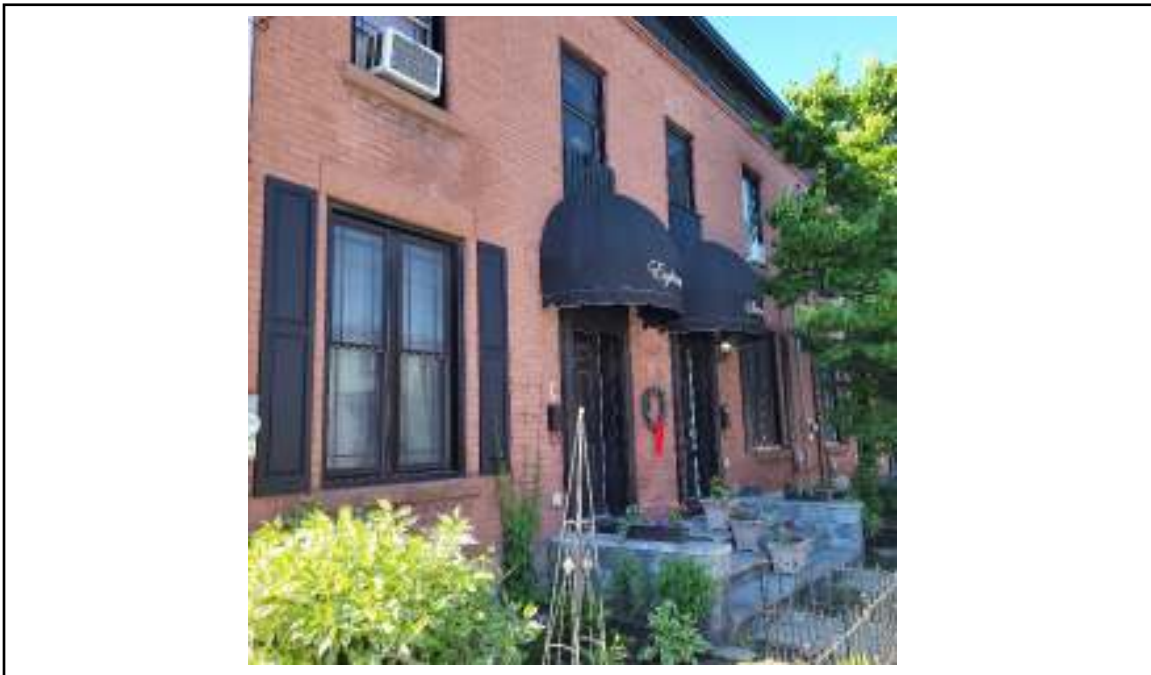
Photograph 1: Looking south-west at north end (front) of 18 and 16 Hawthorne Avenue.
