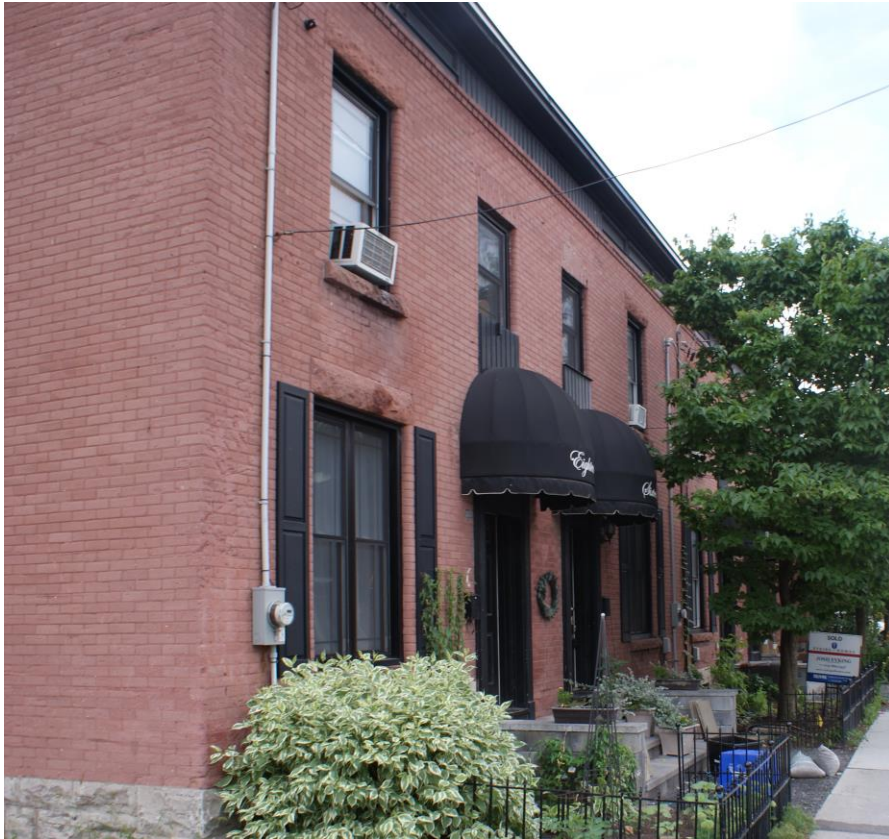
Figure 10: View of the front façade of the townhomes with paired entrances and cultured stone landings and steps. Source: Commonwealth
