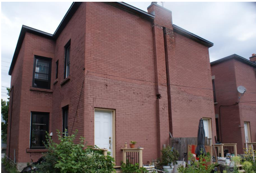
Figure 13: View of the back of the L-plan townhomes set-back to-back forming a T-plan. The roof line of the removed rear porches is evident on the brickwork Source: Commonwealth.
