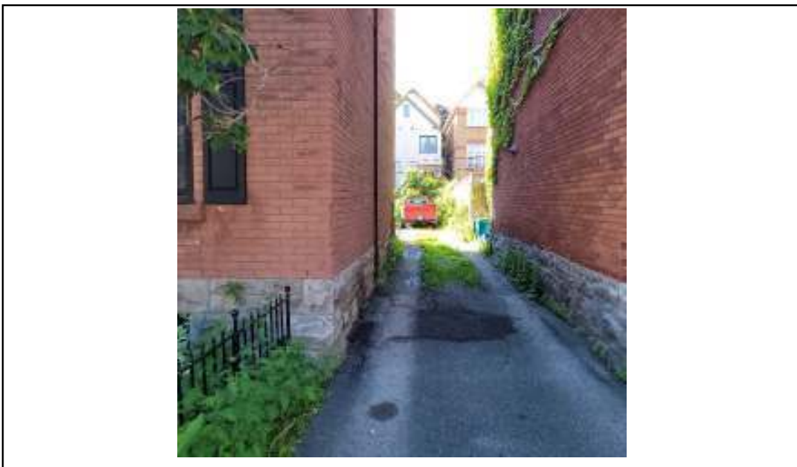
Photograph 30: Looking south from asphalt laneway of 12. Note fill and vent pipes for AST in basement of 12 Hawthorne on brick wall, center of photograph. Off-site property 10 Hawthorne is on left.
