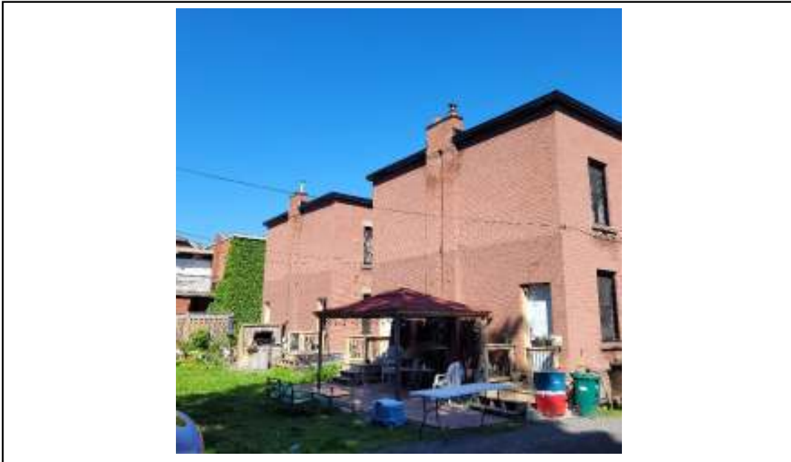
Photograph 25: Looking north-west from south-east end of 18 Hawthorne at back (south end) of buildings.
