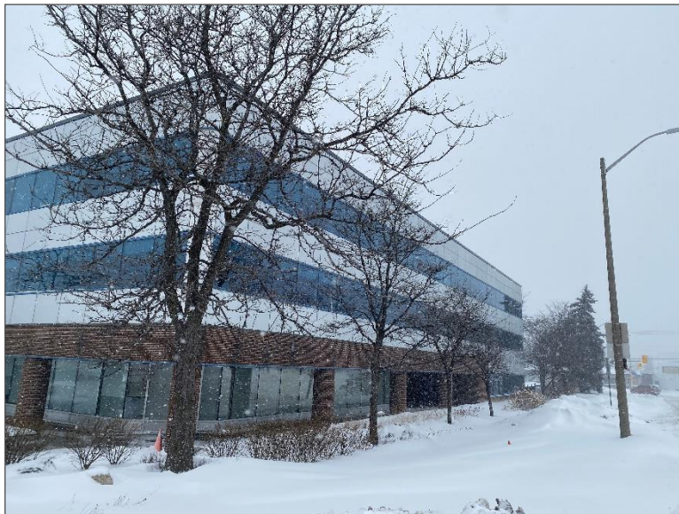
Photo 2 – Site Building (east elevation).
