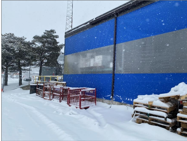
Photo 3 – Site Building (partial view of the west elevation).
