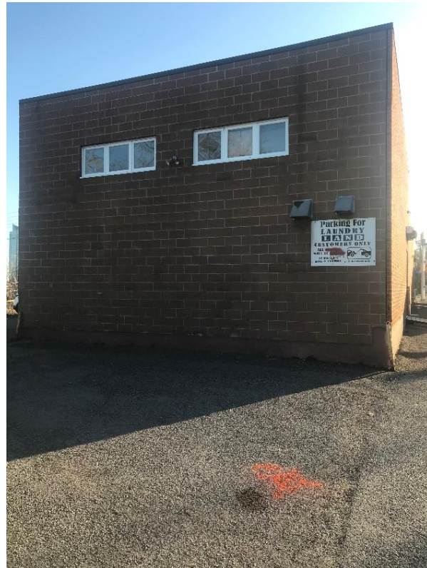
Photograph 6: West face of Site building, facing east (April 6, 2021).
