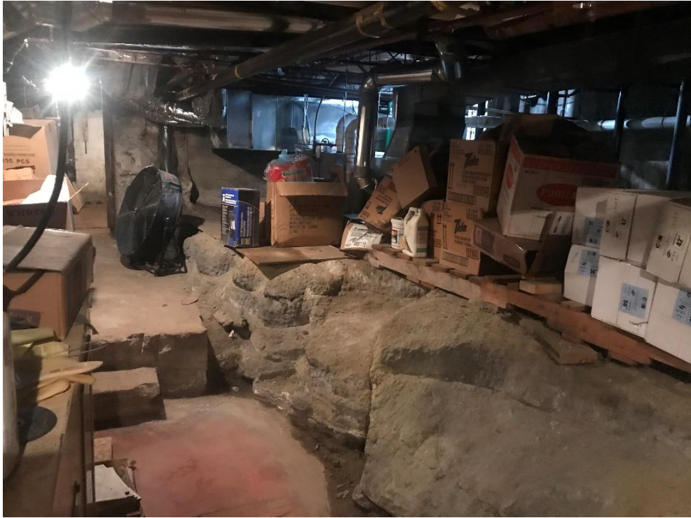
Photograph 21: Site building basement, storage (April 6, 2021).
