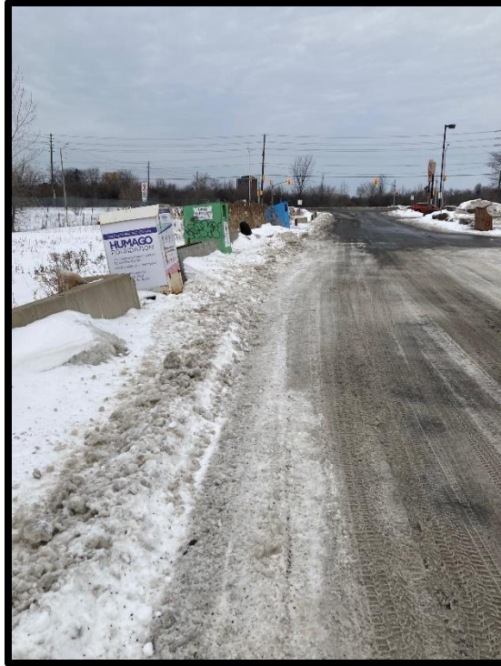
Photograph 3: View of the asphaltic concrete roadway on the 1920 Walkley Road portion of the Phase I Property, facing north.
