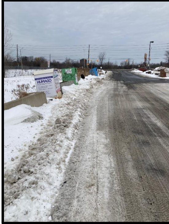
Photograph 3: View of the asphaltic concrete roadway on the 1920 Walkley Road portion of the Phase I Property, facing north.
