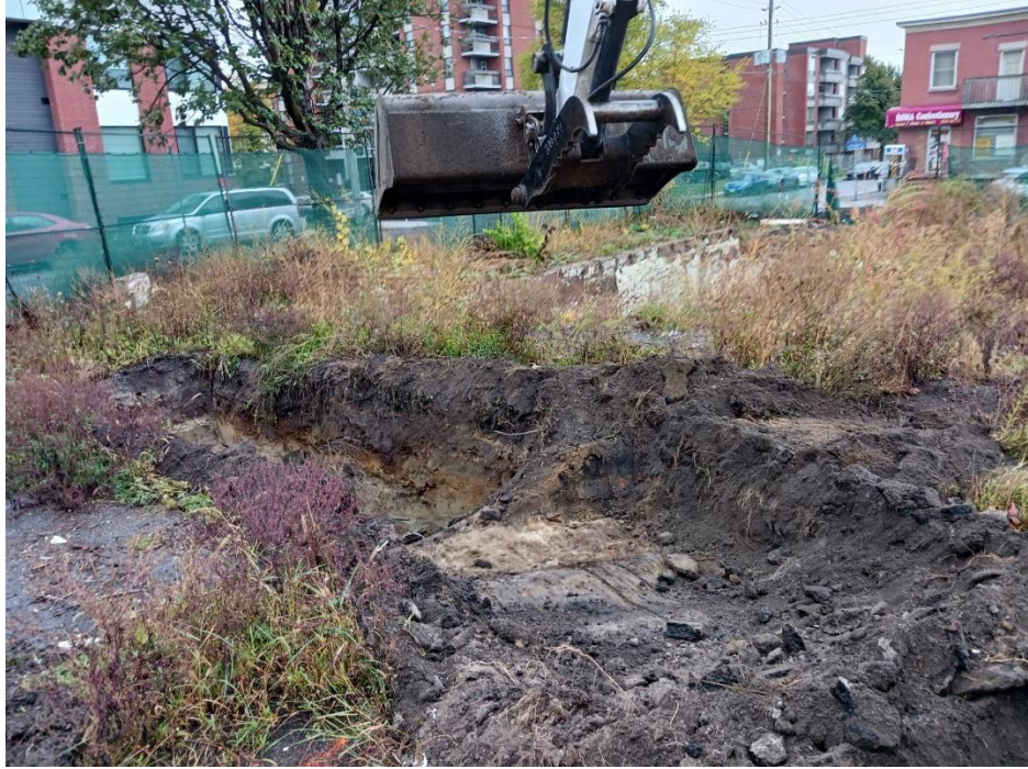
Image of excavation commencing
