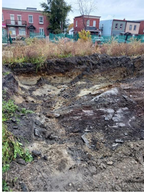
Image of scraped soil exposing lime stone bedrock
