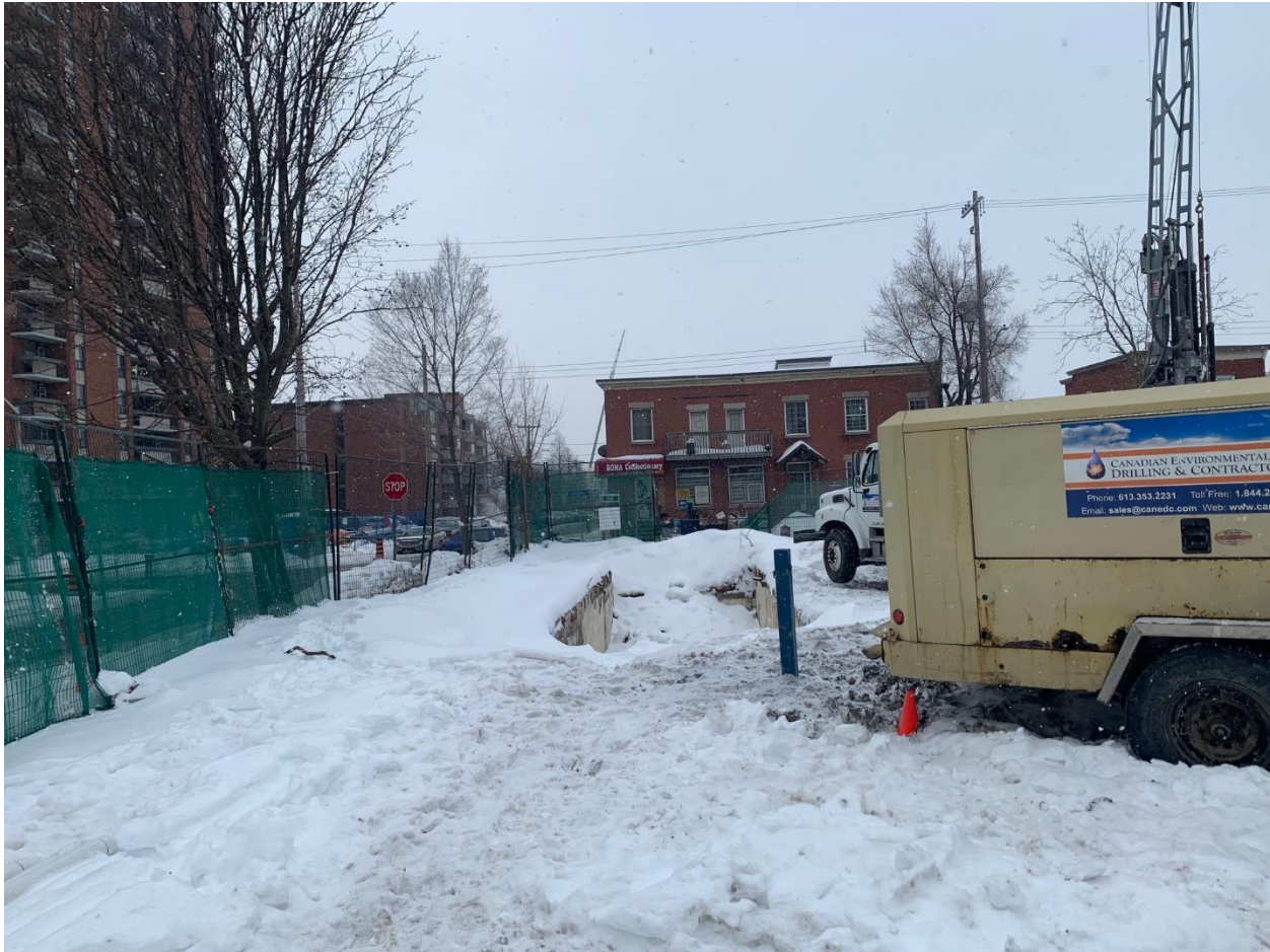
Image 1 – Monitoring Well 4, facing west (later decommissioned)
