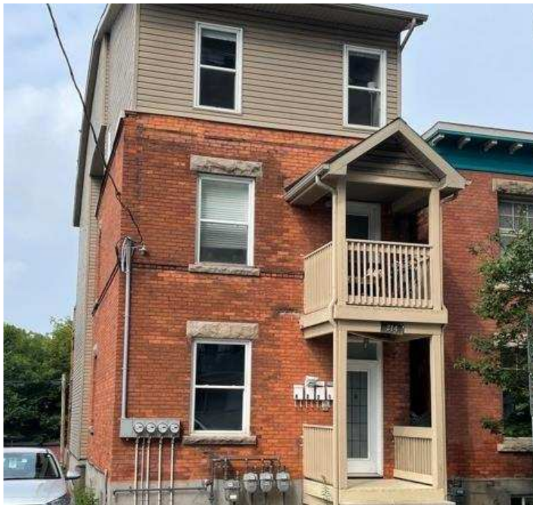
Photograph 1: View of the east side of the subject building, taken from Bell Street South.
