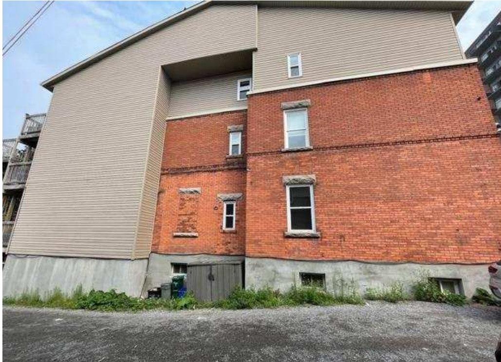
Photograph 2: View of the southern side of the subject building.
