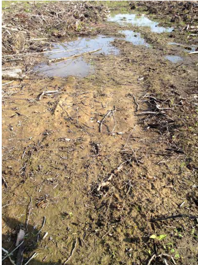
Figure 58: Exposed subsoil after grubbing took place (D374).
