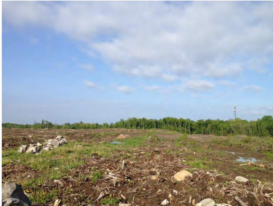
Figure 57: Southern area after grubbing took place (D370).
