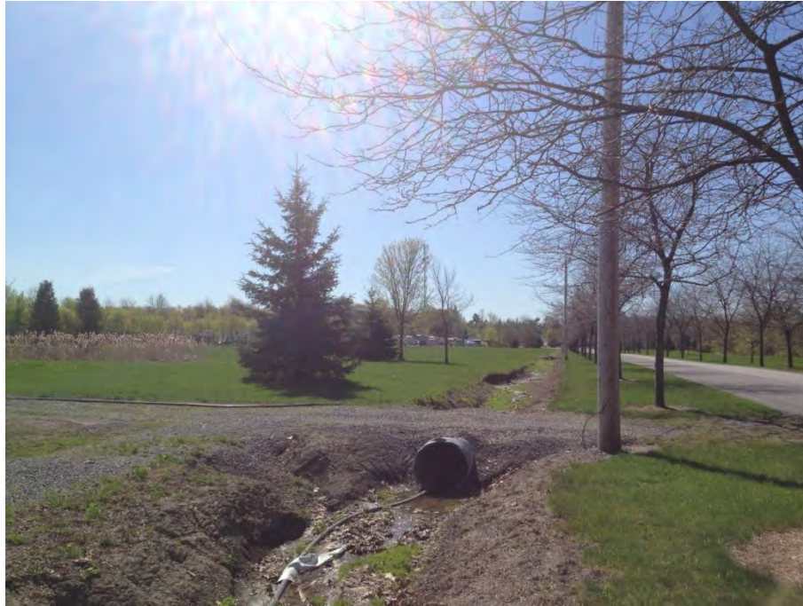
Figure 82: Drainage ditch alongside grassy area and driveway to Laporte nursery (D250).
