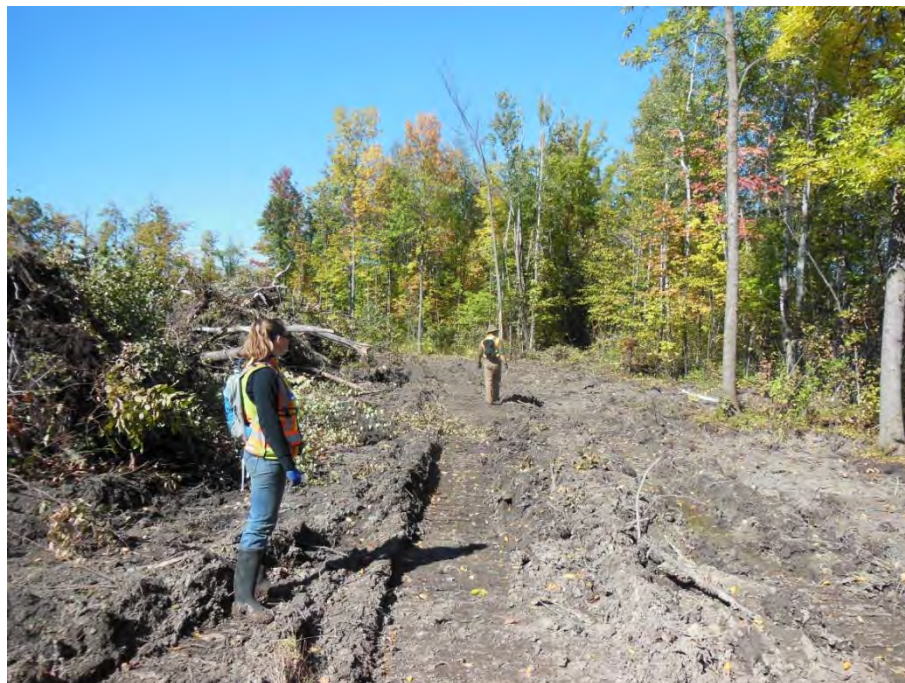
Figure 56: Inspecting grubbed area in Operation 11 (D221).
