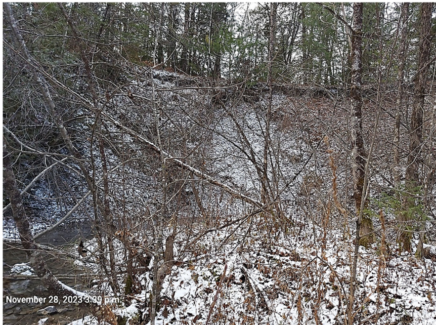
Photograph taken facing the left bank along the upstream extent of R4 . Valley wall contact was observed. Scour, undercutting and woody debris in the channel were commonly observed. The downstream extent of the reach was backwatered due to a second dam at the confluence with Cardinal Creek.
