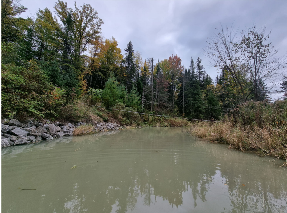
Photograph taken facing upstream at cross-section 5; located upstream of one of three beaver dams observed. Slope stabilization works comprise the right bank around the meander bend for erosion protection.
