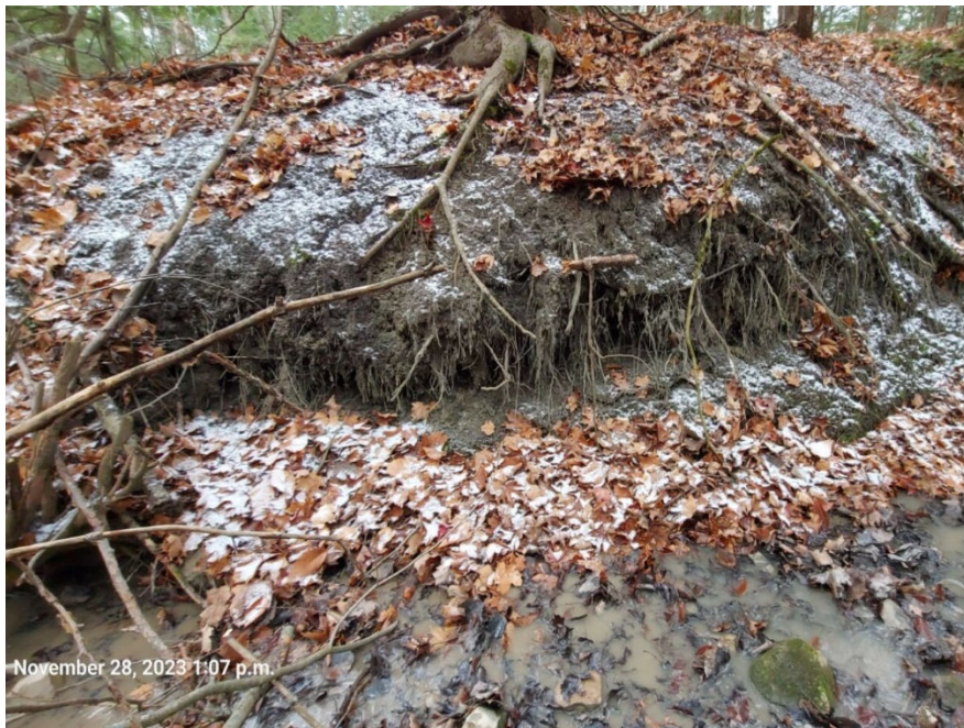
Photograph taken facing the right bank along T1 . Undercutting, exposed roots and woody debris jams were commonly observed.
