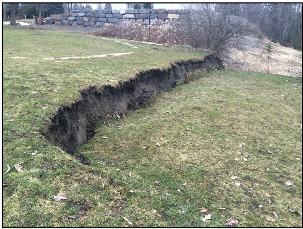
Photo 2: Photograph of failure observed along the top of slope at the property site. Photo taken from the southwest portion of the subject site. Photograph provided by the property owner.
