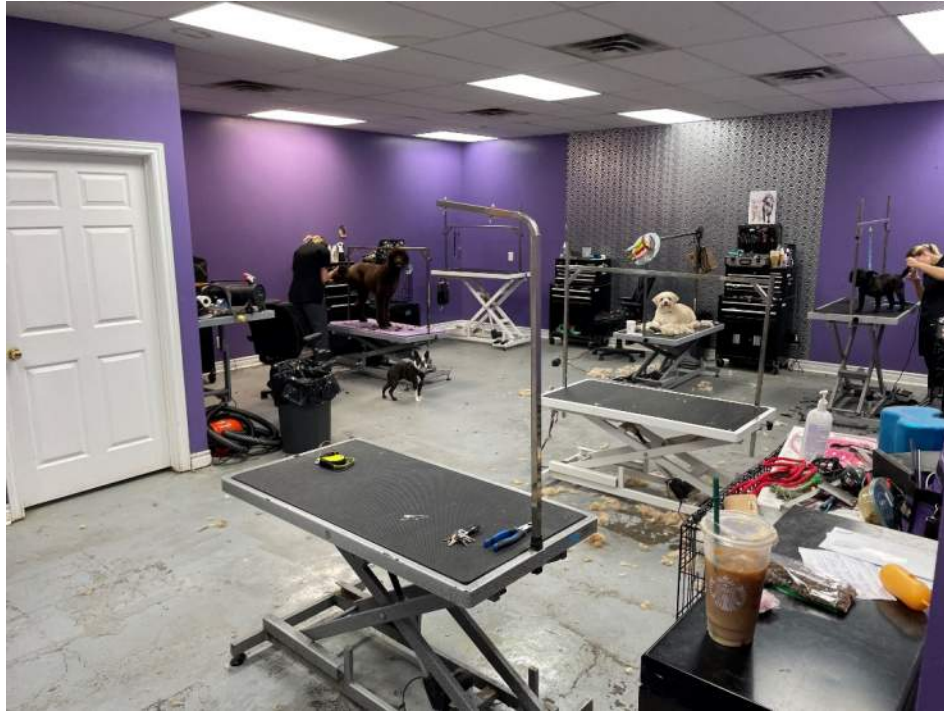
Photo 9: Interior finishes in one unit of 591 March Road.
