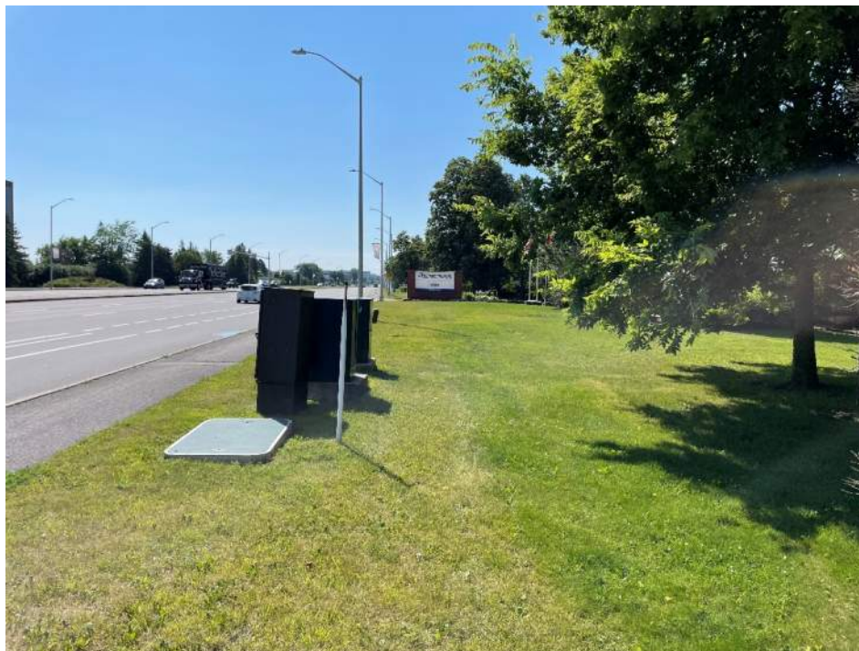
Photo 2: Northern corner of the phase one property looking southeast along property line. Communication pedestals lined up along the side of March Road.
