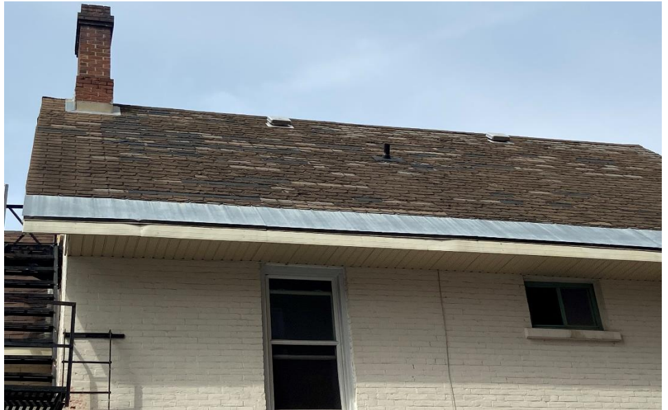
11 Roof and chimney of 230 Lisgar. MTBA
