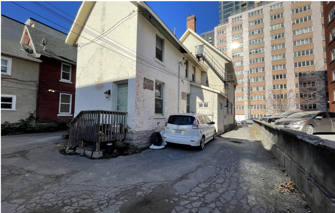
Photograph 4: View of the 230 Lisgar Street, looking northwest
