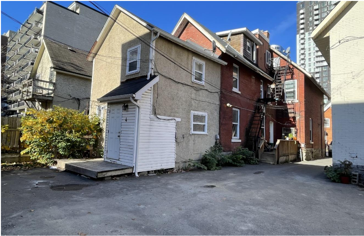
Photograph 3: View of the 232 Lisgar Street, looking northwest.
