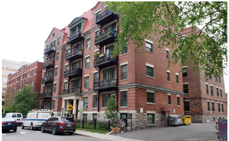
45 The Shefford, designated under Part IV of the Ontario Heritage Act. MTBA
