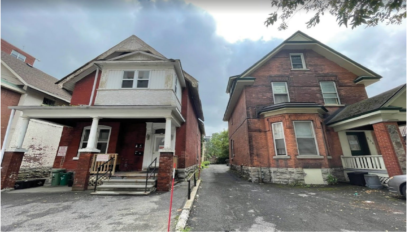
Figure 5: Subject site (232 Lisgar Street to the left) and neighbouring property (to the right), looking south
