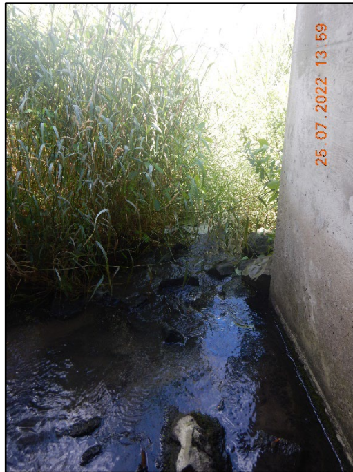
3. Wilson Cowan Drain - Facing downstream from inside culvert, the flow path is to the right side of the culvert flowing into a defined channel
