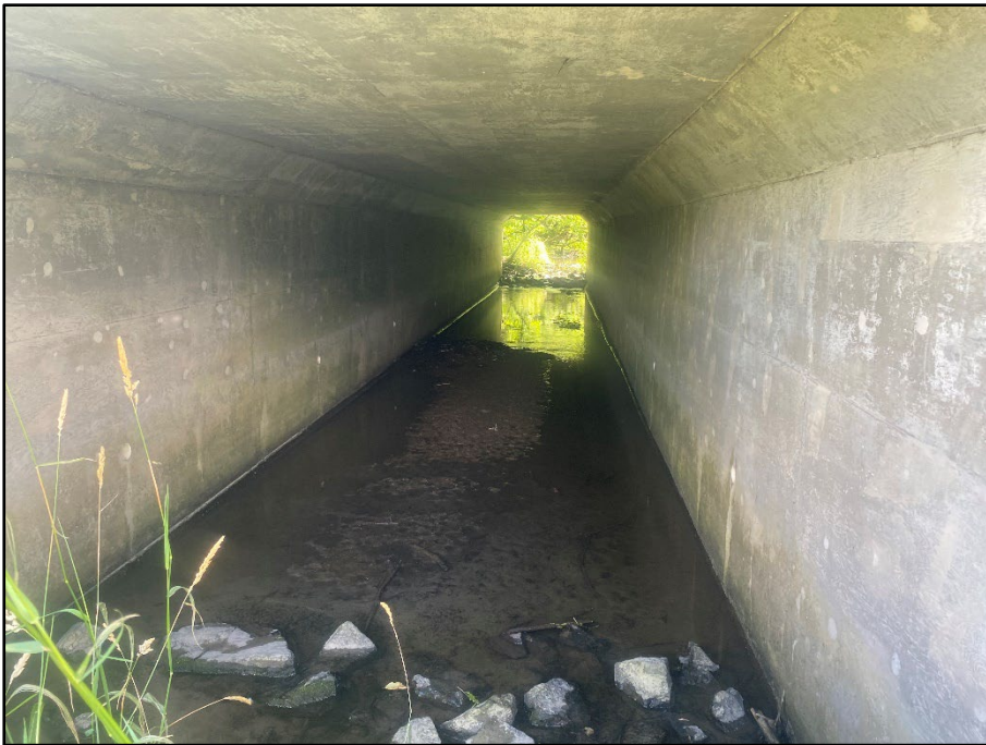
2. Wilson Cowan Drain - Facing upstream from outlet of culvert passing under Bankfield Road
