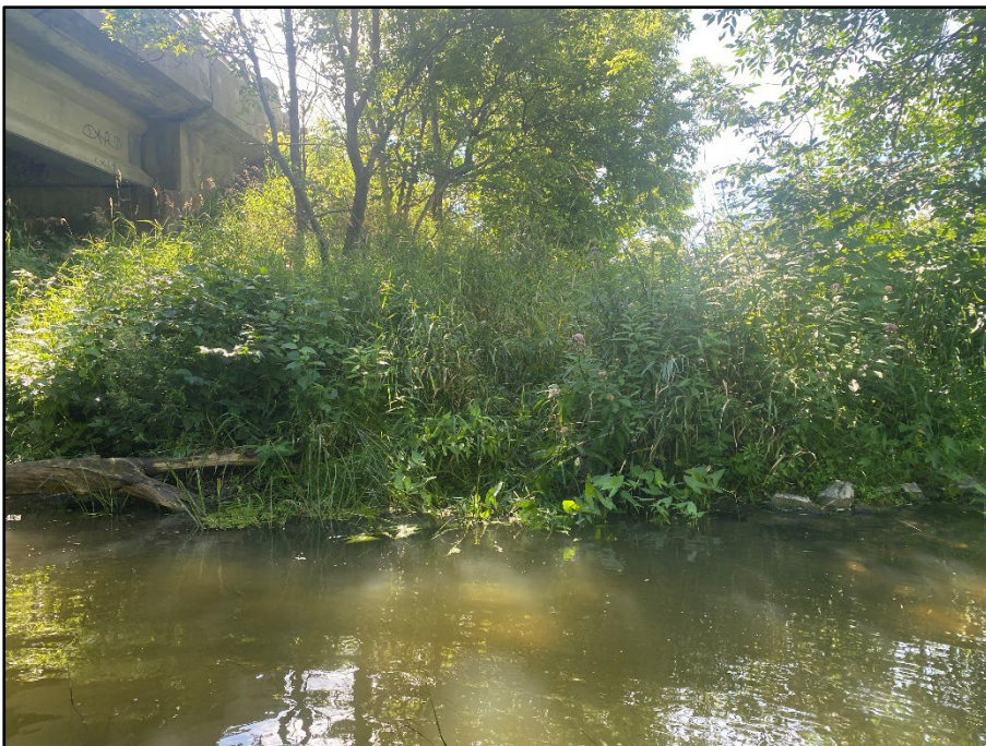
10. Mud Creek – Facing parallel to Rideau Valley Drive N, inlet location from the Oxbow feature into Mud Creek with an approximate 1 – 1.5 m elevation change
