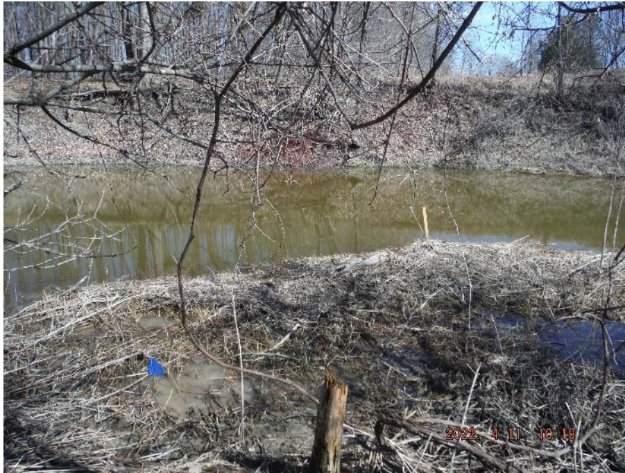
Photo 16: Looking at the steep bank along a portion of Mud Creek that is on Site (April 11, 2022)
