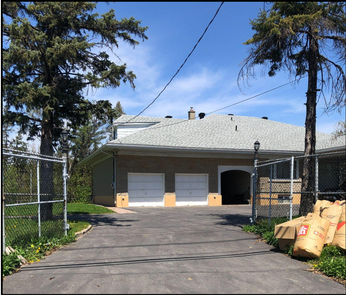
Existing building (front facade) at 1765 Montreal Rd.
