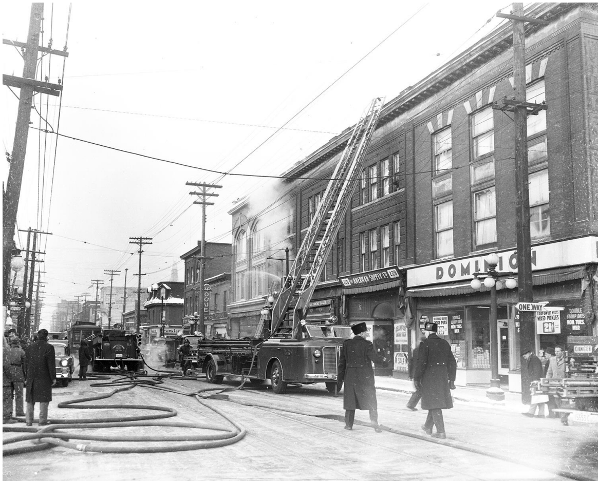
Figure 17: A view of the 211-231 block with fire trucks in the street. Note the unpainted facades with the decorative keystone with spandrels between the 2 nd and 3 rd floors. The photo provides a record of the earlier retail storefronts.
