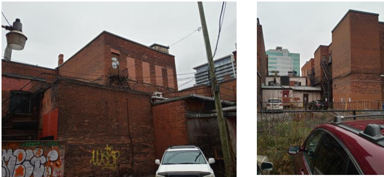
Figure 16: Views of the east facades (rear).
