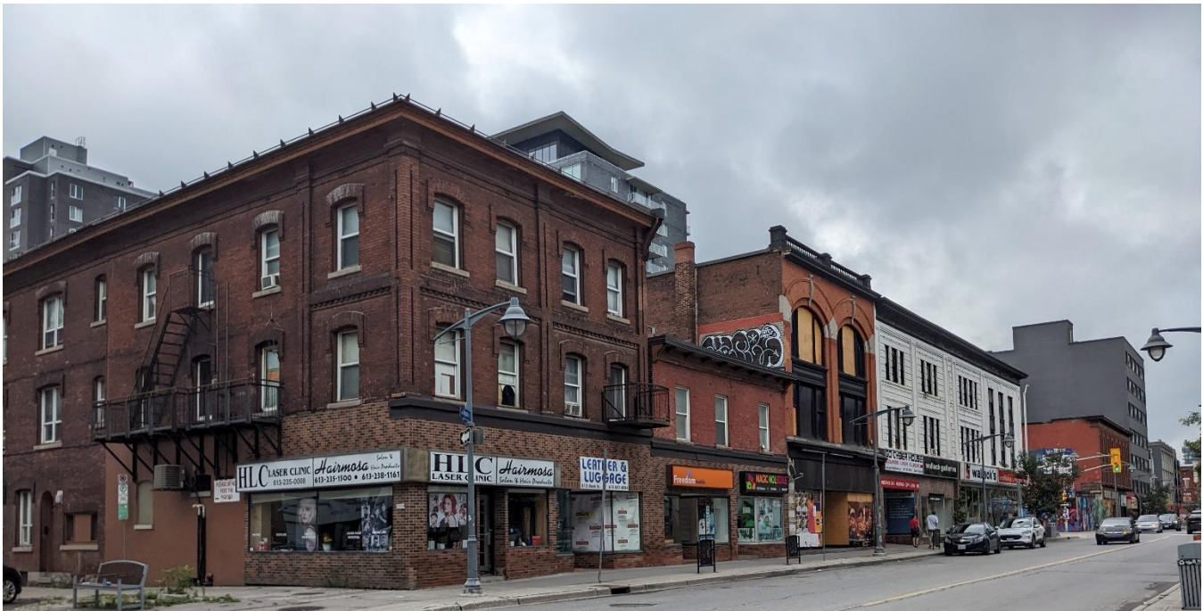
Figure 1: Subject Property, looking south-east at Existing Buildings
