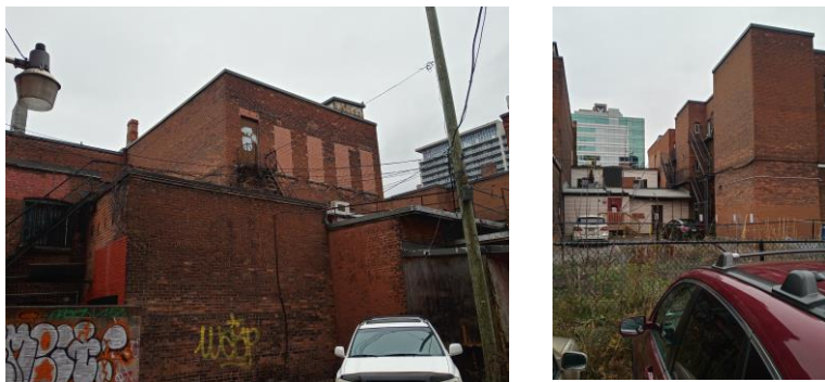
Figure 16: Views of the east facades (rear).
