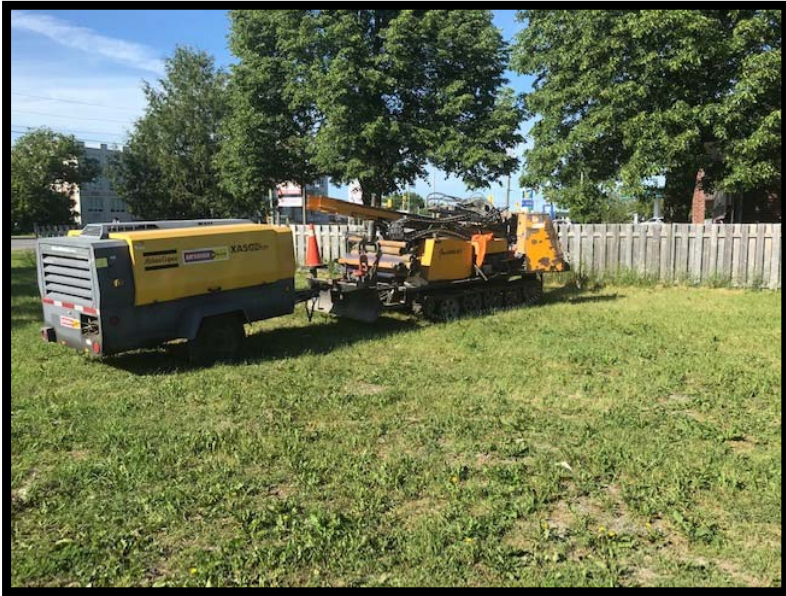
Drill Setting Up at MW1 – June 19, 2020
