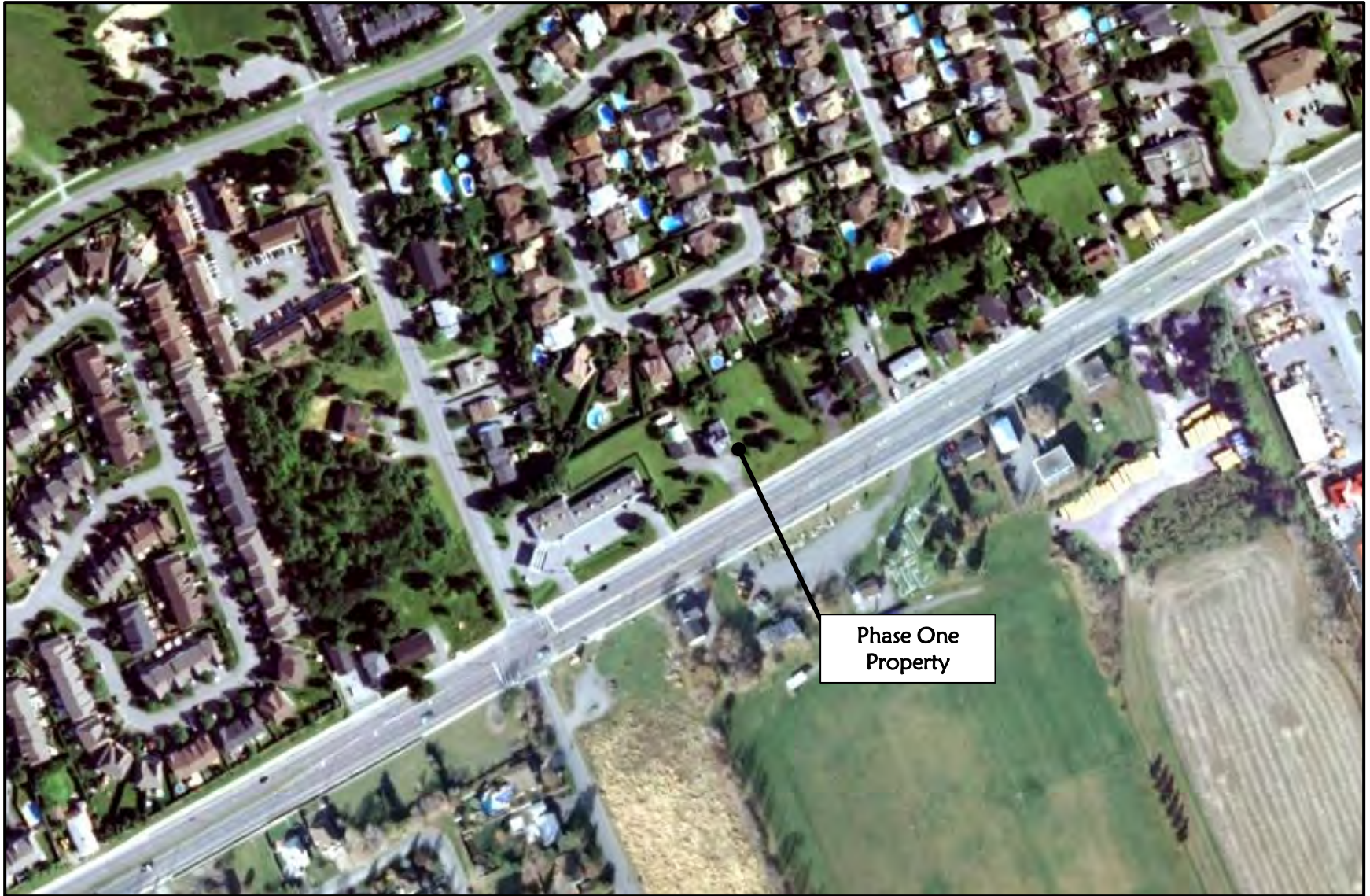
Historical Aerial Photography of the Site 3493, 3497, and 3499 Innes Road, Ottawa, Ontario 2008 230028 – January 2023
